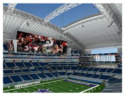
extrusions in the massive end-zone door, as well as over 30 miles of aluminum louvers on the exterior. The giant screen hanging over the field stretches from one 20-yard line to the other, and weighs as much as a 747 aircraft.
